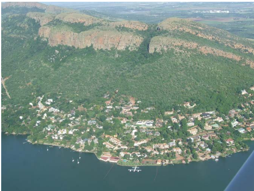
AERIAL VIEW OF THE HARTBEEPOORTDAM WHICH IS 10 MINUTES FLIGHT AWAY FROM WONDERBOOM AIRPORT
